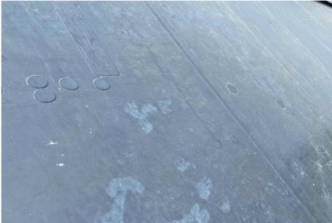
Figure 3. Seven patches in this area – Material 1.1mm, Age approx. 3 years.
