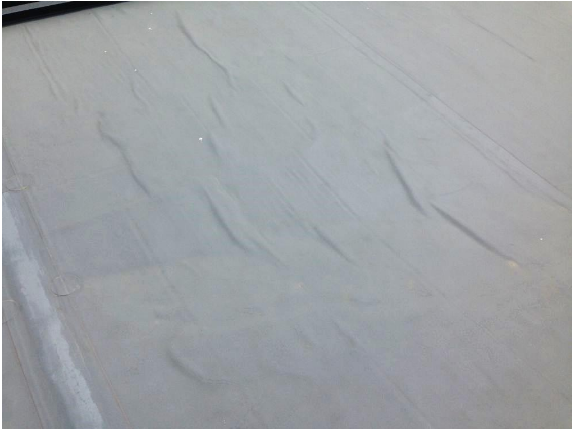
Figure 5. Three patches (of 6 on the roof). Material 1.2mm, age 2 years
