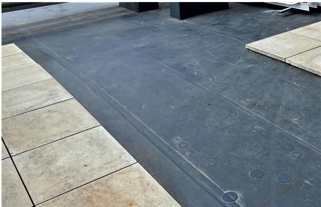
Figure 4. At least 12 patches in this area - Material 1.1mm, Age approx. 3 years.
