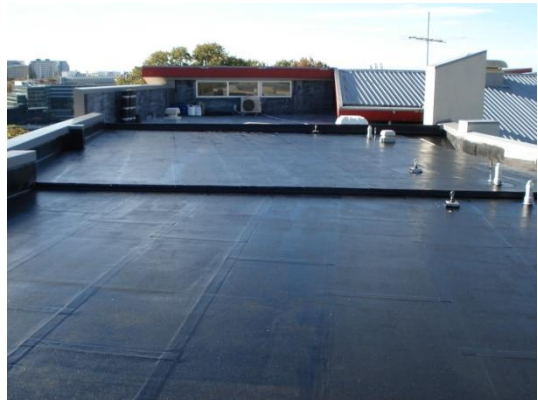
Cleaned and Primed
