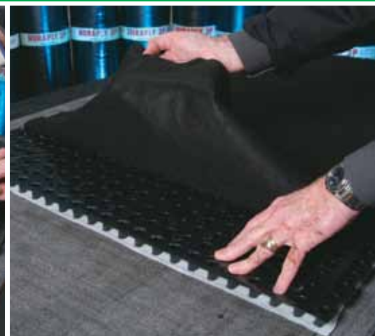
Drainage mat laid on membrane
