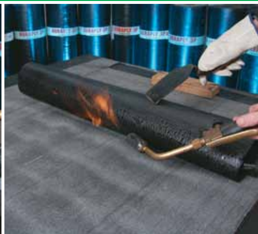
3PG heat welded to basesheet
