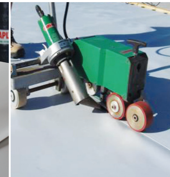
C - Welding sheet joints
