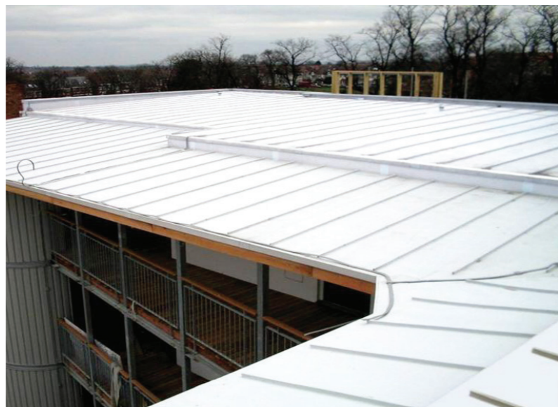
Belgium Nuratech with Batten Detail
