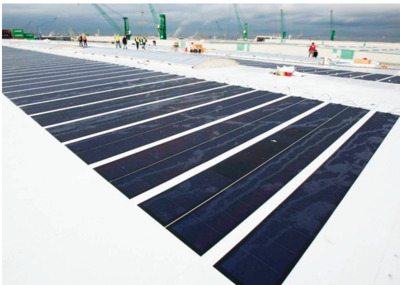
Nuratech membrane with NuraSolar Panels installed
