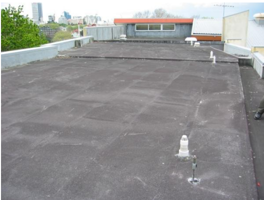
Roof in Original Condition
