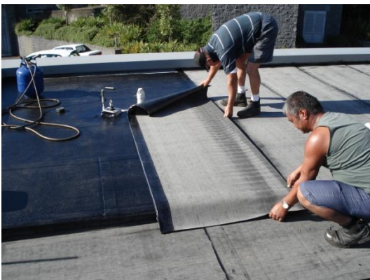
Measuring out new membrane
