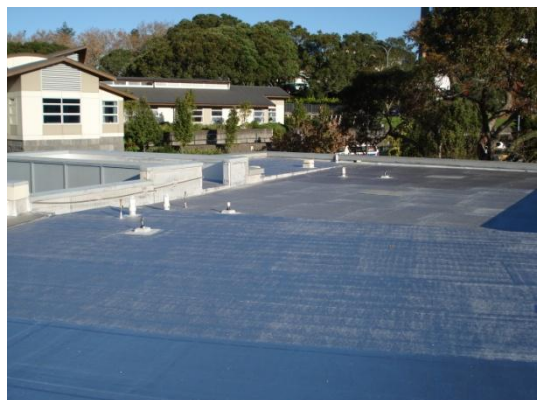
Completed overlaid roof
