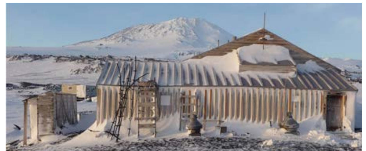
» Scott's Hut, reroofed by Cheshire Architects
