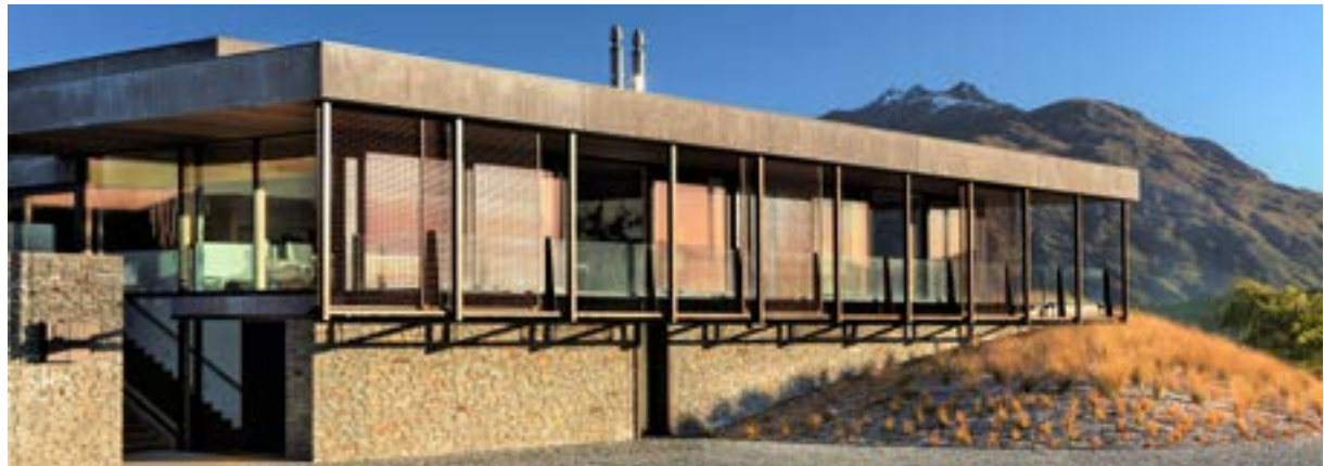
» Oliver's Ridge by Team Green Architects
