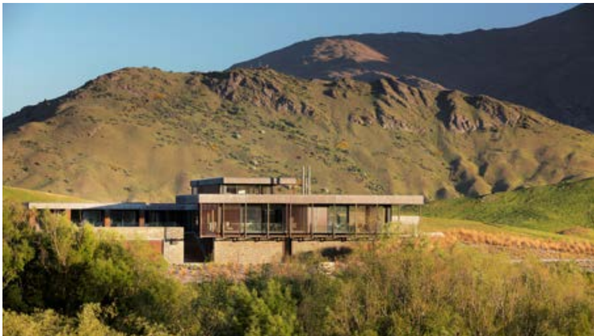
» Oliver's Ridge by Team Green Architects
