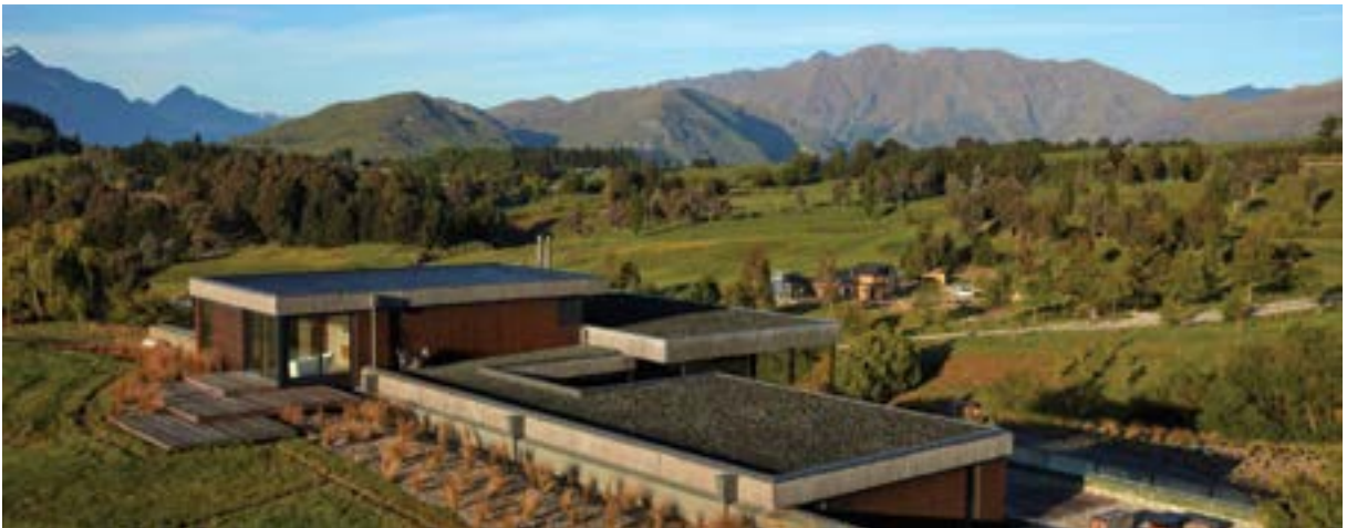
» Oliver's Ridge by Team Green Architects
